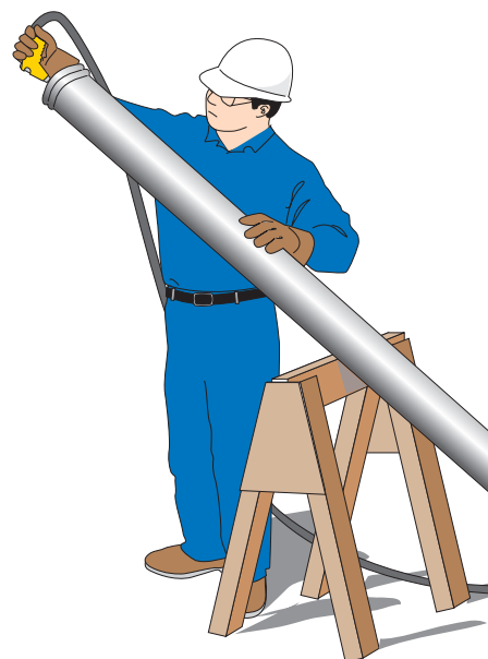
Figure 14 Washing the Pipe System
