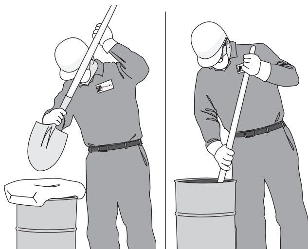
Figure 16 Mixing Slurry in a Barrel
